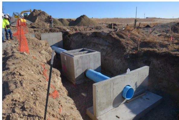
41A-3-6 Long Crested Weir Inlet/Drop off in progress
