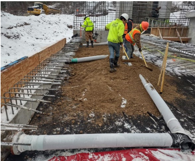
Jacko K Canal Diversion Dam & headworks reconstruction began in September 2022
