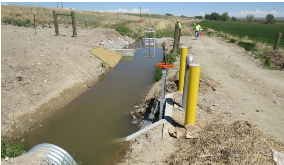
Completed 41A-3-6 Long Crested Weir Inlet/Drop
