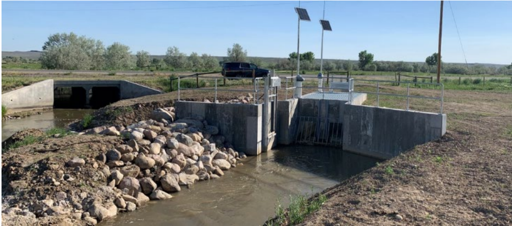
Completed 14B-44 Construction on Point of Diversion
