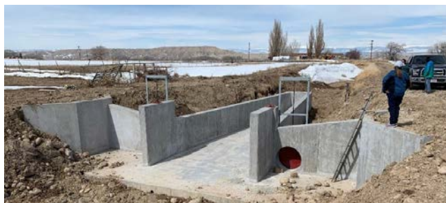
Shephard's Check under construction
