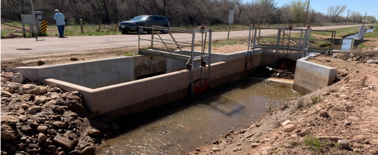
Bench Canal, Bottle Hollow Splitter new construction in operation
