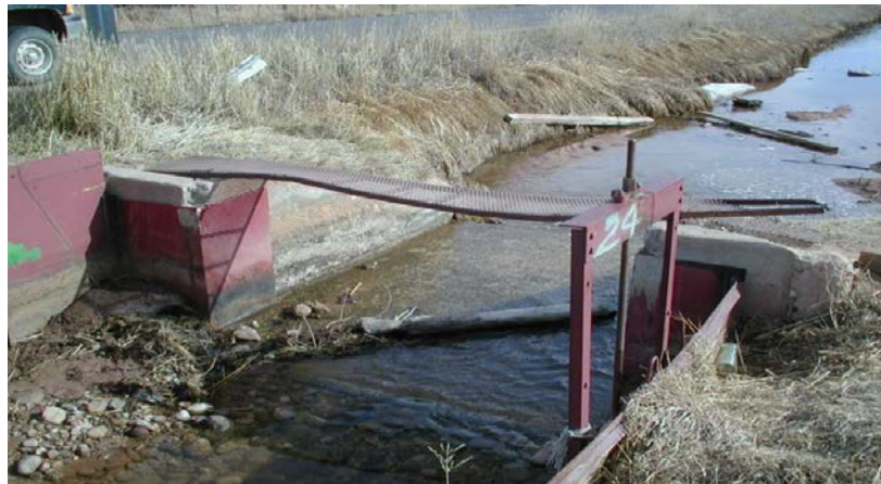
Bottle Hollow Check prior to rehabilitation
