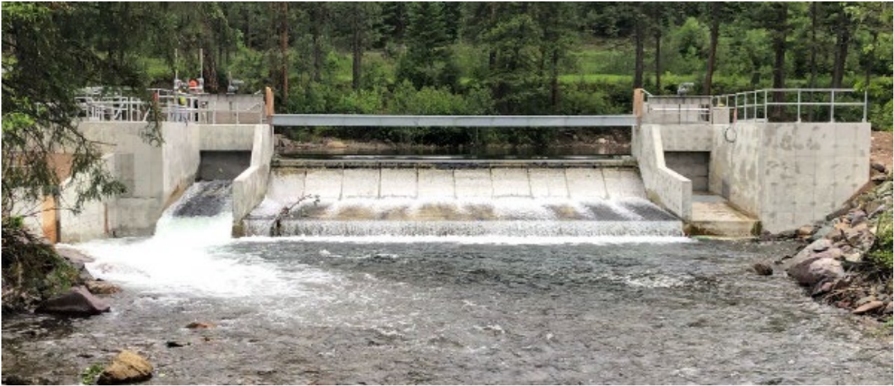
Jocko Canal after Restoration
