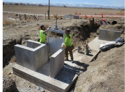
Wind River Irrigation Project reconstruction, 41A-3-6 Long Crested Weir Inlet/Drop off construction in progress
