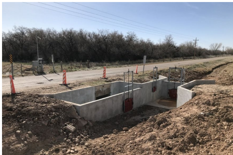
Bottle Hollow Splitter under Construction
