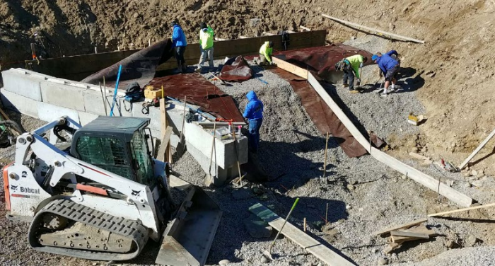
Wind River Irrigation Project reconstruction, 41A-3-6 Long Crested Weir Inlet/Drop off construction in progress
