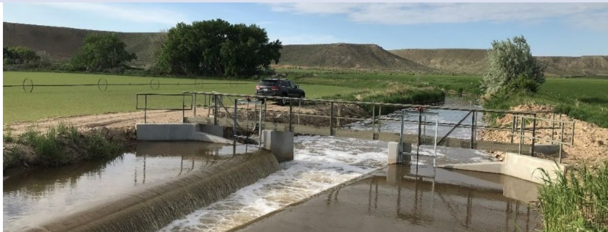
Gray Mountain Canal, Shephard's Check new structure in operation
