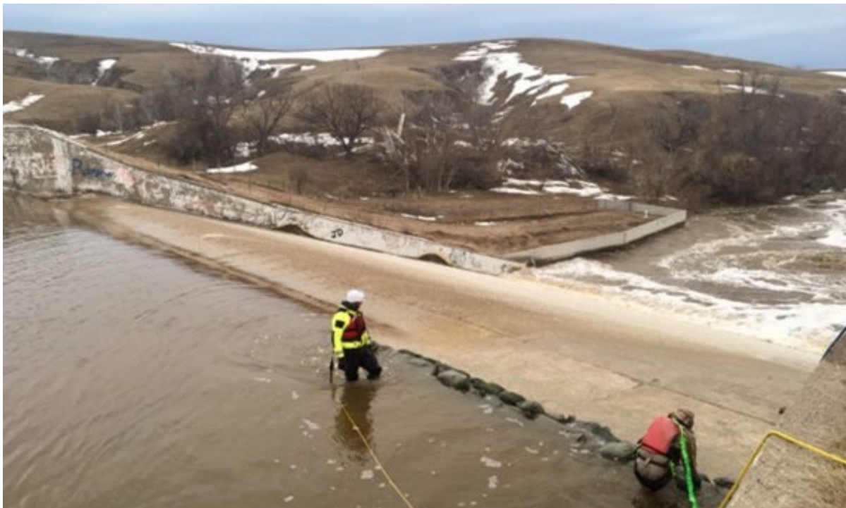
Dam Safety staff sandbagging the Oglala Dam spillway during the 2019 flooding.
