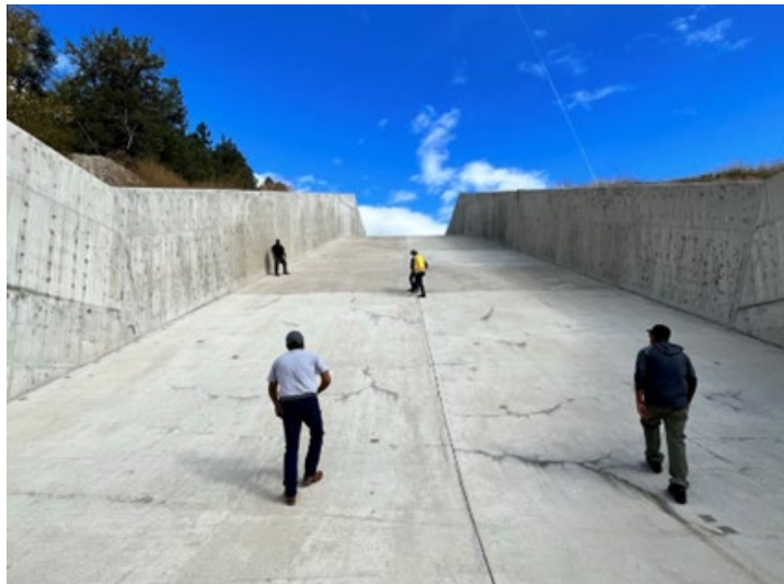
Dam Tender Training attendees perform a mock inspection Crow Dam's concrete spillway on the Flathead Reservation in Montana.
