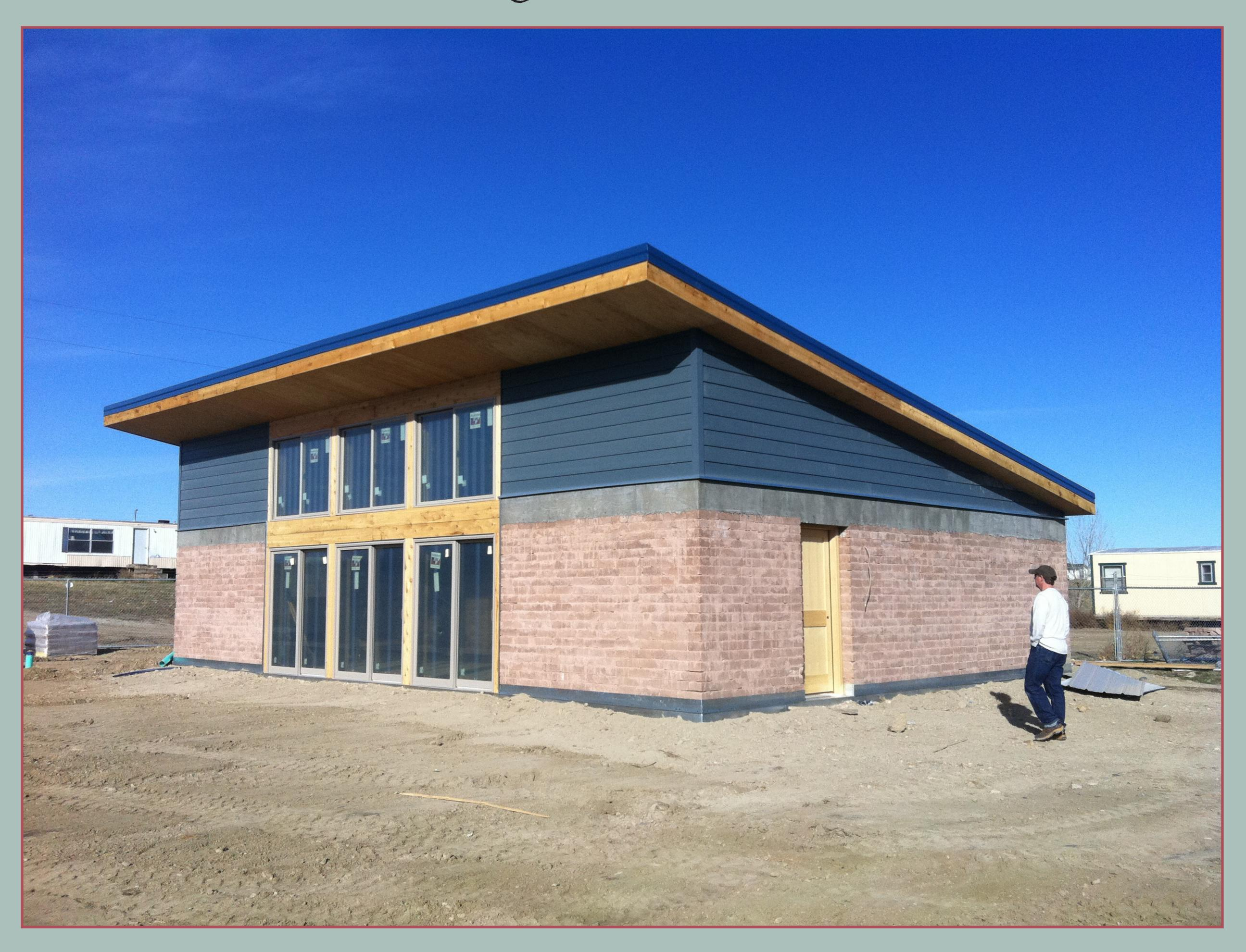
Each home site is carefully oriented with southern exposure, a specially designed foundation, and geothermal heat pumps to maximize energy efficiency
