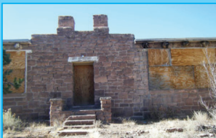
Building 401 is an example of stone structures on the Hunters Point Boarding School campus. It was built in 1935.
