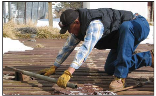
Smith struggles to open a water turn-off valve outside the BIA Roads Maintenance building at the Mescalero Agency. The valve wouldn't budge.
