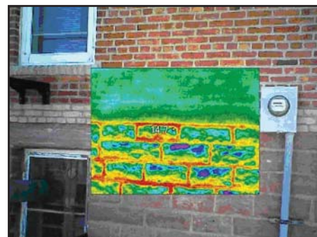
An infrared photo of the foundation of the Flandreau administration building.
