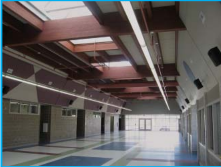
Interior daylighting at St. Francis Indian School helps save energy by reducing the need for electric lighting.
