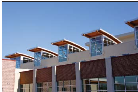
The Sac and Fox Tribe and OFMC shared in the cost of constructing the Meskwaki Settlement School. The tribe also will fund part of the O&M for the replacement high school in Tama, Iowa, which will be dedicated this summer. These clerestory windows are part of the school's LEED-inspired design to add daylight.
