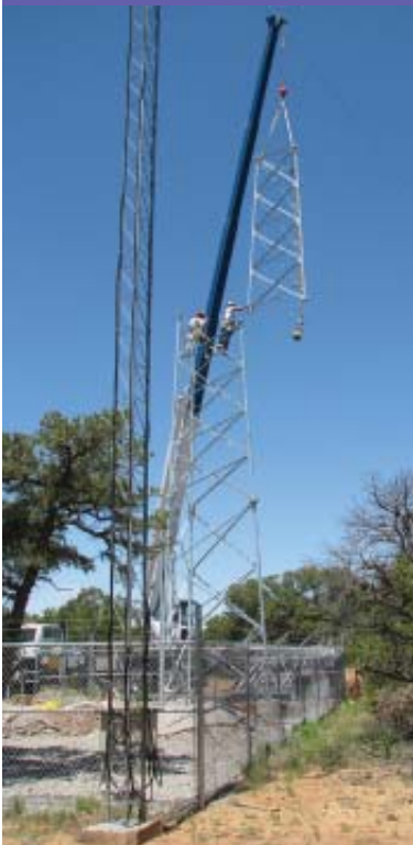
While the old tower is still in service, a new communications tower serving Zuni Pueblo is erected. See Page 3.
