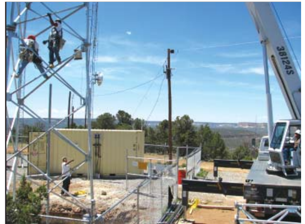
On a ridge overlooking Zuni Pueblo in New Mexico, workers assemble the new communications tower, which has a more substantial base (below left) than the old tower (below right).
