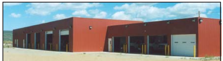
The new Navajo Region Wildlands Fire Management Shop-Vehicle Storage Building in Ft. Defiance, Ariz., is based on a standard design developed by former Southwest Region Facilities Architect Robert Clayton. Similar buildings are used by BIA agencies at Taos Pueblo, Zuni Pueblo, the Mescalero Apache Tribe, and other federal agencies around the country.
