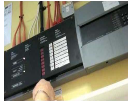
Testing the fire alarm system
