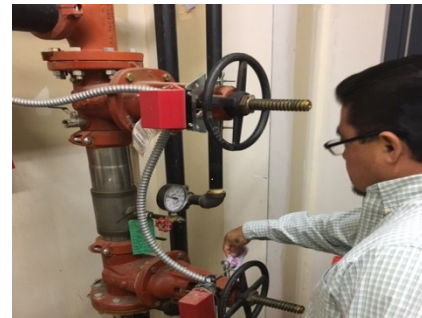
Central Office Annual Workplace Inspection by DSRM Inspector
