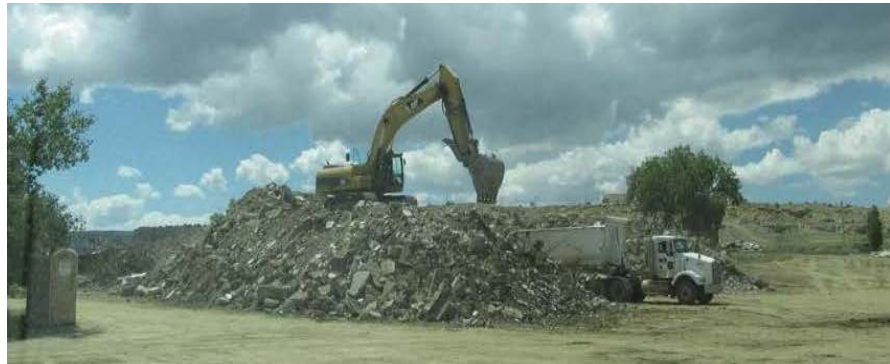
Demolition of Crown Point Boarding School, NM.
