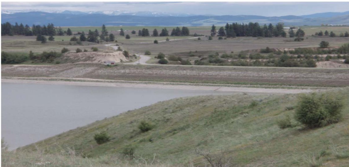
Crow Dam, Flathead Indian Reservation, Montana
