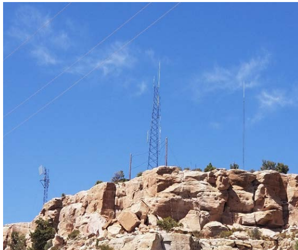
Telecommunications Tower, Keams Canyon Arizona
