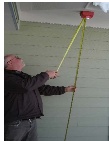
Facility Condition Assessment, Ute Mountain, Towaoc Colorado
